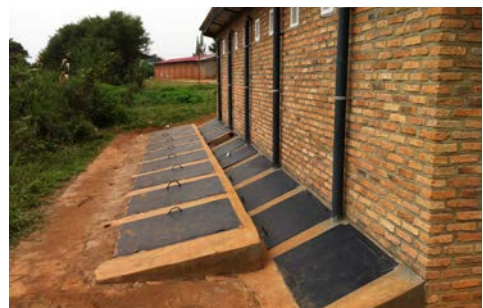
Fig.3.35 Compartment to Separate Human Waste in EcoSan
